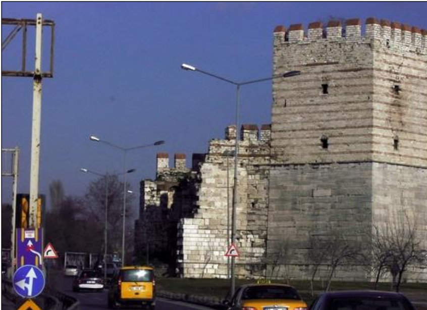
Figure 1: Existing Kennedy Caddesi Near Marble Tower Structure
